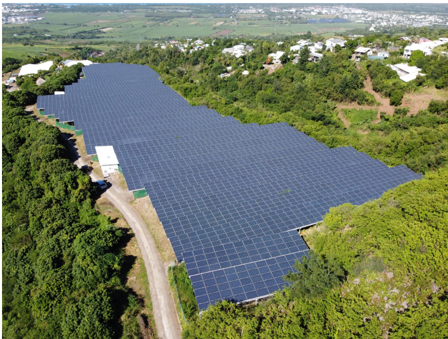
The Domaine de Bellevue agrivoltaic power plant, 2.5MWp
